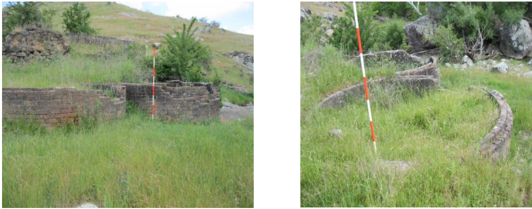
Figure 14a Showing two historical circular brick tanks at the complex.
