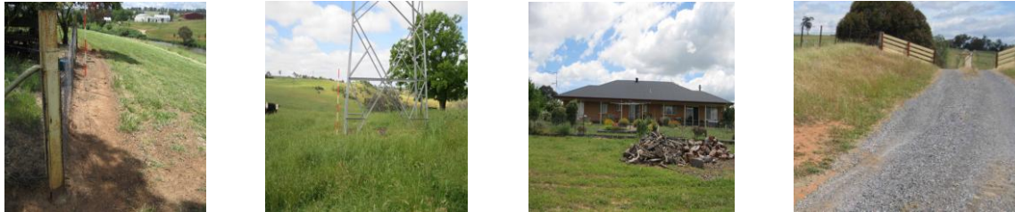
Figure 7 Some past ground disturbing activities at the study area, from left: fence line, steel power poles, house construction, and road building.
