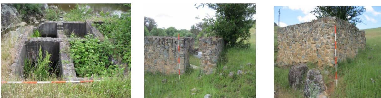
Figure 14 Showing some of the brick and stone historical features at the complex.
